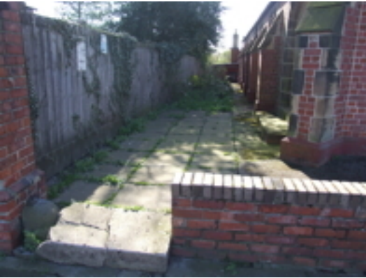
Paving to eastern boundary to north end
